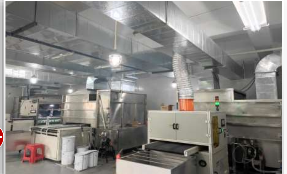
5 FULLY AUTOMATIC FUEL INJECTION LINES
